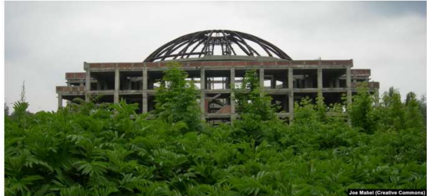
A 2006 photo of an unfinished hunger circus in the southwestern Rohava neighborhood that was later demolished to make way for a shopping mall.
